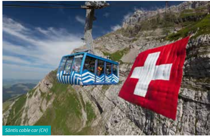
Säntis cable car (CH)
